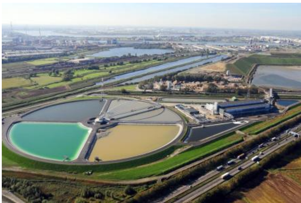
Figure 11. Treatment of Contaminated Dredged Material 5
