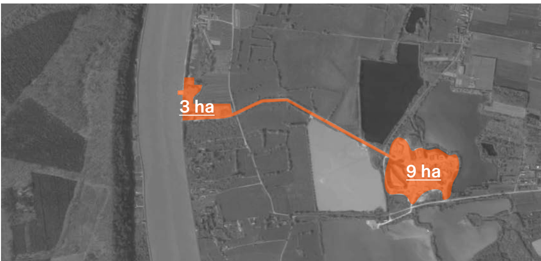
Aggregates quarry of Cemex company and its transhipment platform implanted along the Seine, between Le Havre and Rouen
